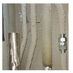
thickness is 1-3 mm dry film. The insulating compound's excellent adhesiveness means that it affixes securely to the underlayer and can also be coated with most paints.
